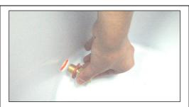
Insert close nipple through the inside of water cooler
